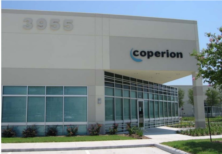
Coperion Corporation – Houston office with sales and engineering capacities.
